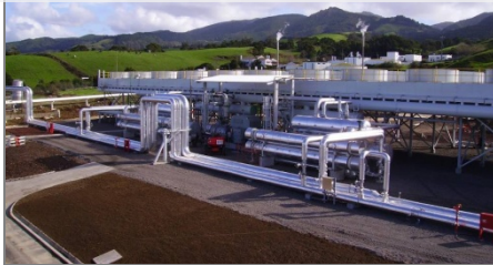
10 MW Geothermal modular binary unit, San Miguel Island
